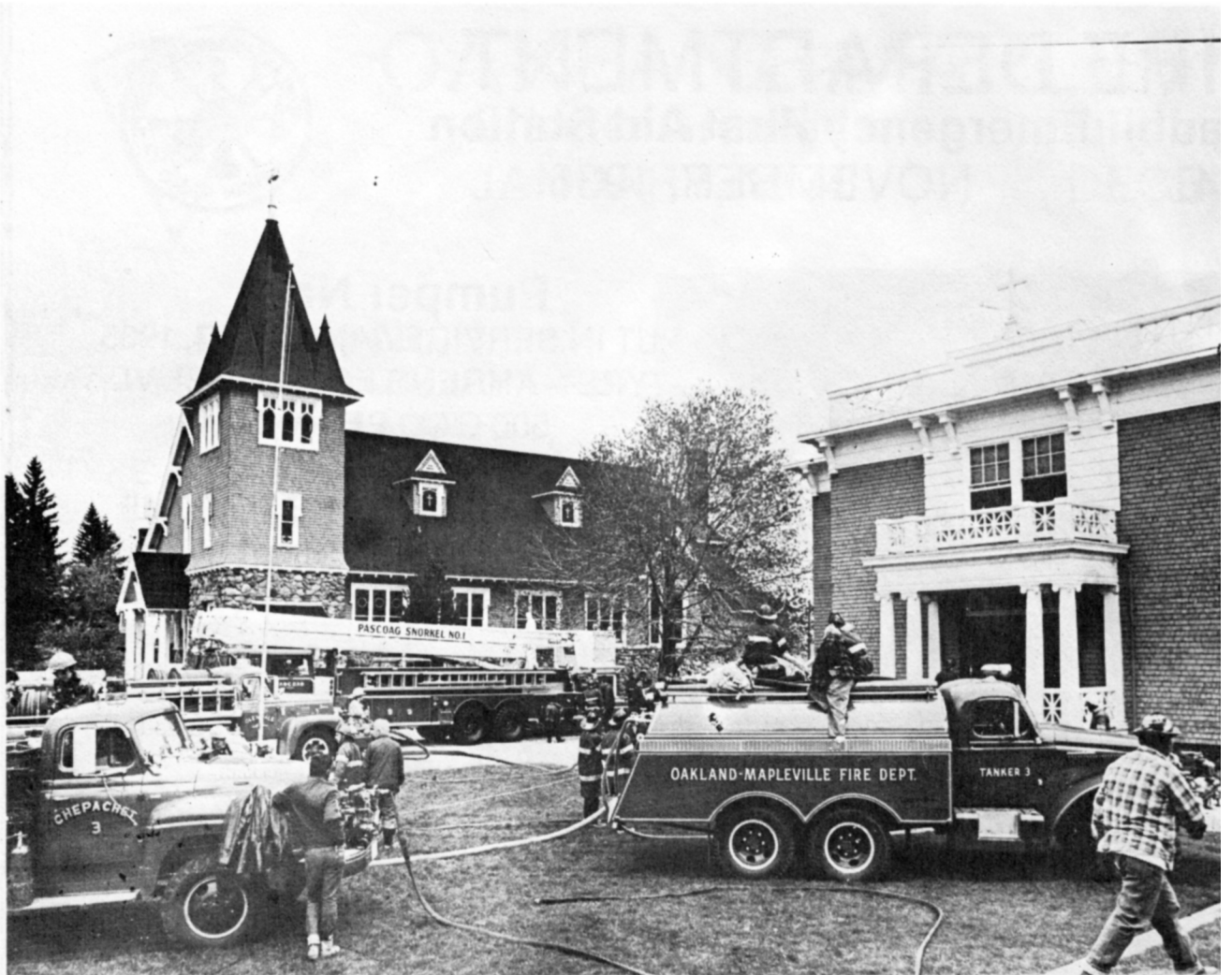
Circa 1971: Tanker 3 at Our Lady Of Good Help School Fire. 1942 International all wheel drive, 1400 gallon tank, 500 gpm pump, built by Ray Balcom, Ed Bertholic, Barry Guston, George Mathewson, Nel Champeau and Ken Brand.
