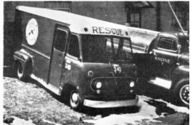
MARCH, 1971 Original Rescue and Engine 3
